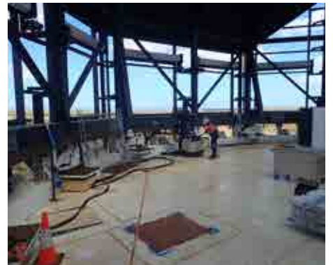
DOME UNDER CONSTRUCTION
