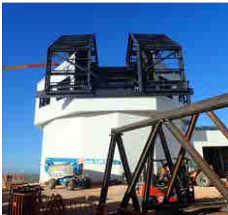
SHUTTER DOOR INSTALLATION
