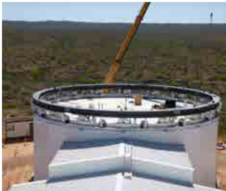
GANTRY RING AND BOGIE ASSEMBLIES INSTALLED
