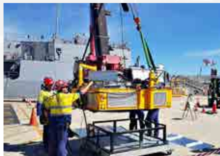
PREPARING FOR THE LIFT
