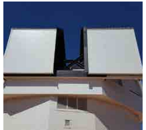
SHUTTER DOORS INSTALLED & OPERATIONAL
