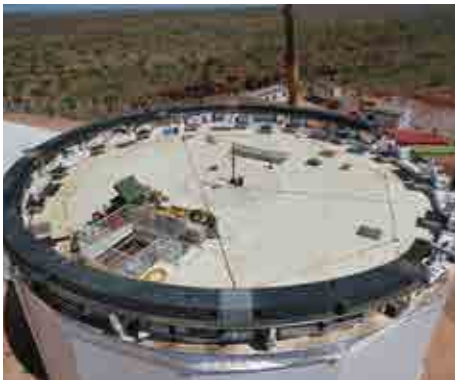
GANTRY RING INSTALLATION
